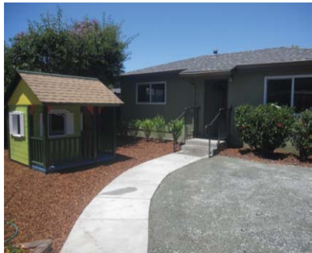
Back cottage after rehabilitation
