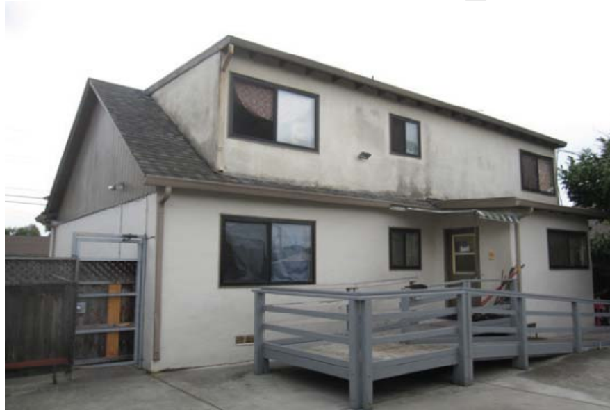
The back of the shelter before rehabilitation
