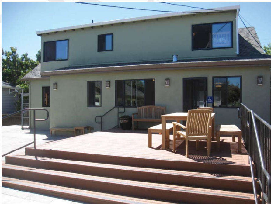
The back of the shelter after rehabilitation
