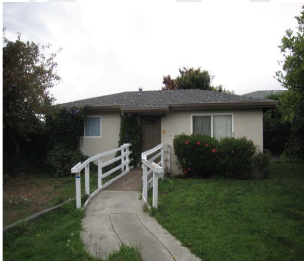
Back cottage before rehabilitation
